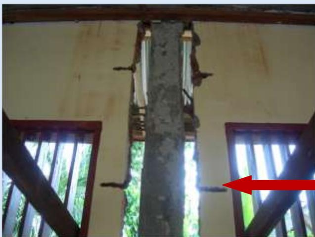
Openings in the side of the wall to insert horizontal reinforcement in the walls which will provide support to the walls
