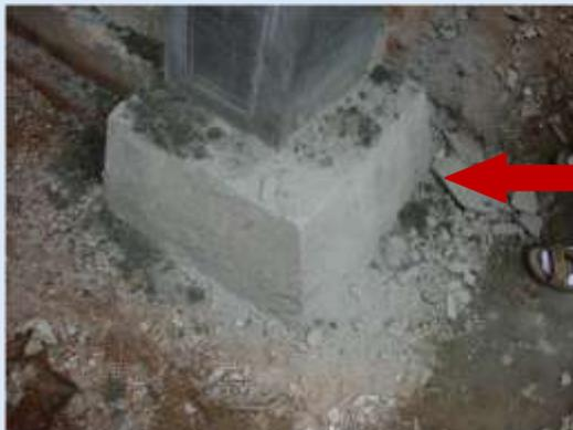
Completed foundation work for a corner column.
