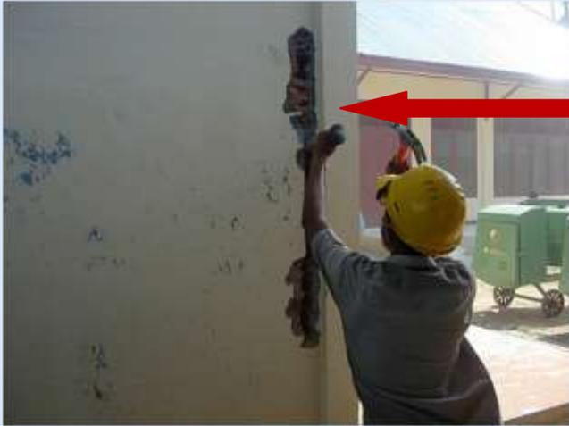
The sides of a column are being opened for jacketing the corner column
