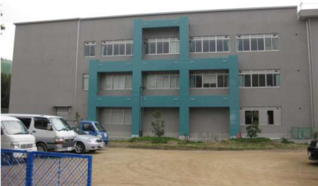
Figure 3-3 Introduction of a steel frame in existing RCC frame building
