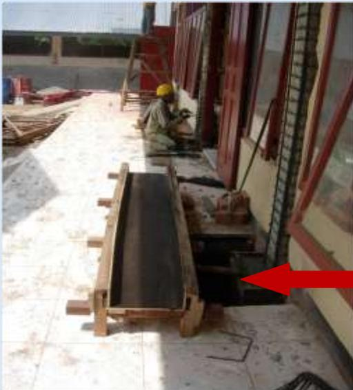
Similar is the case for formwork. A conventional formwork may not be suitable to cast concrete around an existing column and two halves as shown in the photographs may be required.
