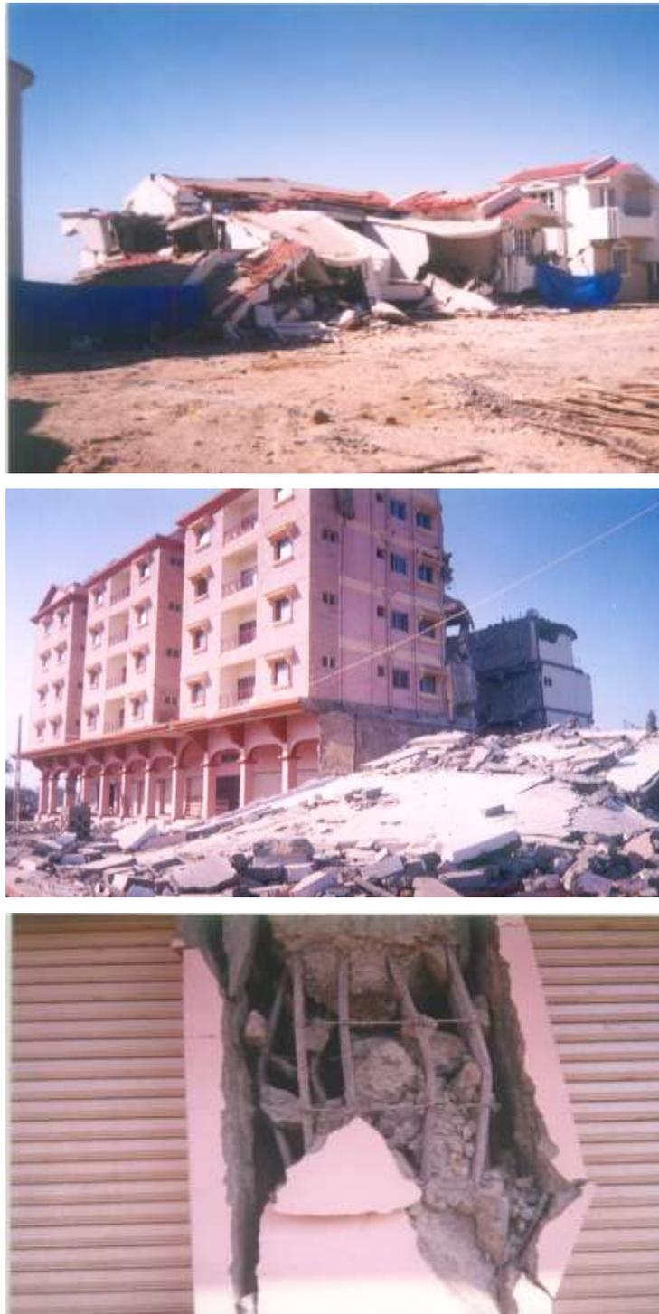
Figure 1-2 Failure of buildings in earthquakes. Beautiful buildings do not mean that they are safe (upper figure). A RCC building failed because of improper positioning of hook reinforcement (below two pictures).
