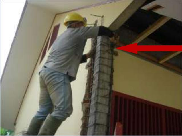
Reinforcement placed in a corner column.
