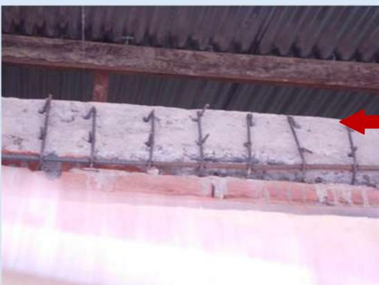
Like in column, complete loop rings are not possible to insert in the beams. U-shaped rings with proper connection may be suitable and engineer should decide on type of bars and rings
