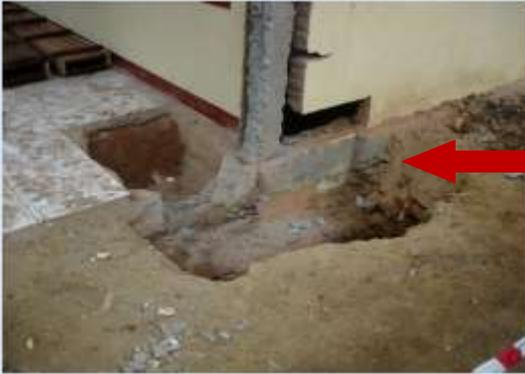
In order to increase size of the footing and also to increase depth of footing, the foundation is opened. The process can be carried along with column jacketing, if necessary
